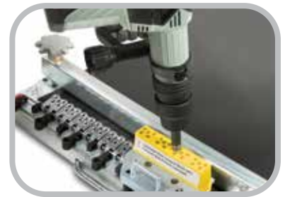
Electric Powered Rivet Driver Installation
