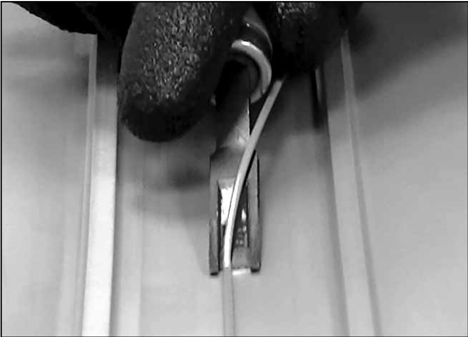
Remove underside weld bead with skiving tool.
