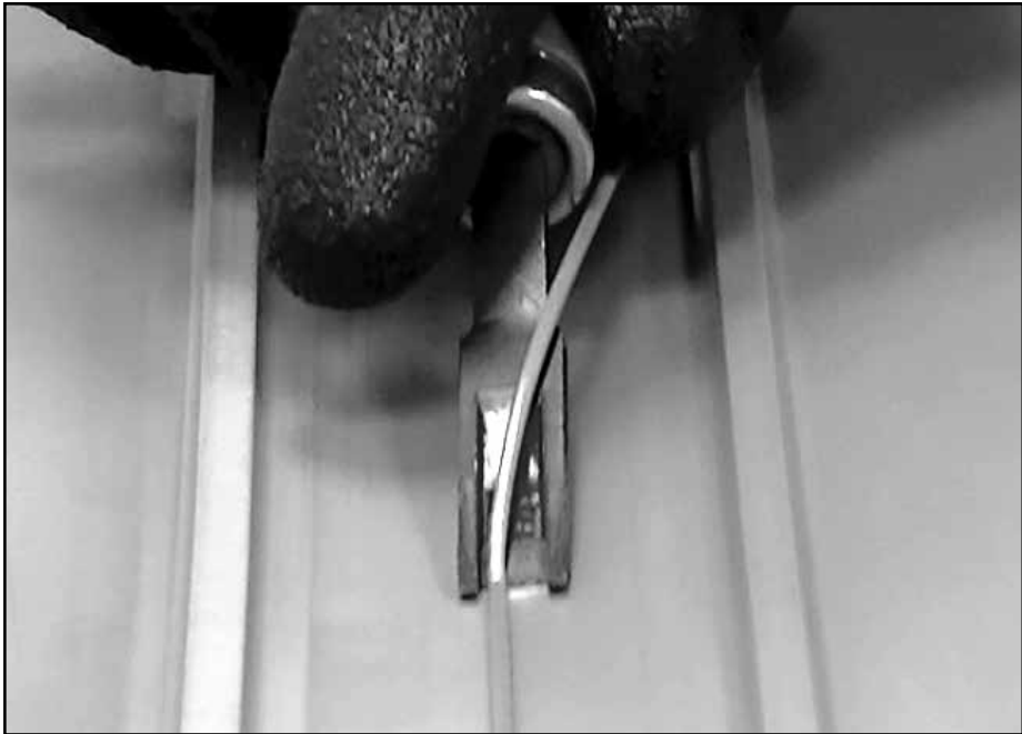
Remove underside weld bead with skiving tool.
