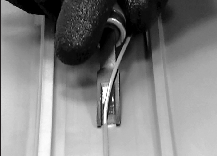
Remove underside weld bead with skiving tool.
