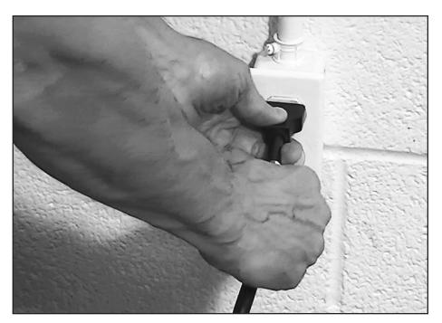
Connect power cable to supply power outlet.
