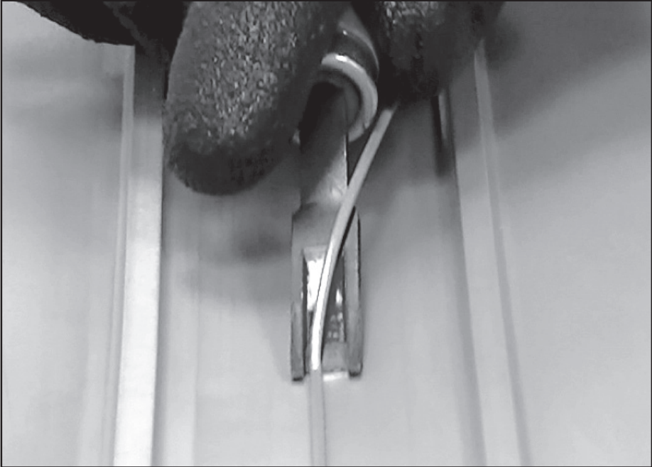
Remove underside weld bead with skiving tool.
