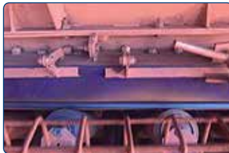
Figure 2: Flexco skirting after 5 days of trial.
