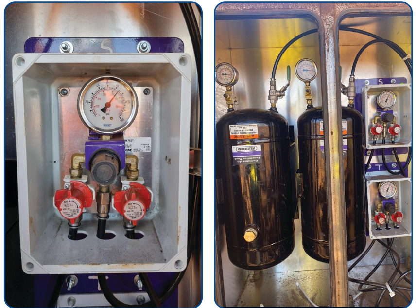
The PAT System Control Box and Tank to monitor the air tension.
