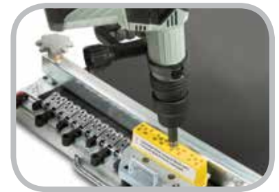
Electric Powered Rivet Driver Installation
