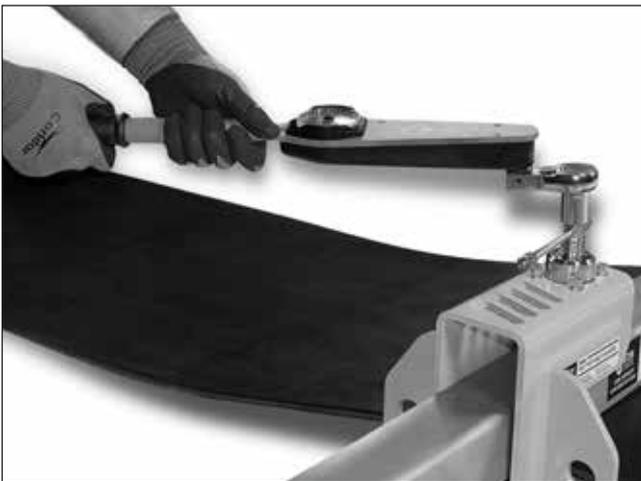
5. Use torque wrench to apply the correct torque value to the clamp end screws.
