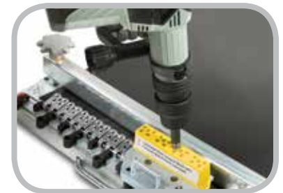
Electric Powered Rivet Driver Installation
