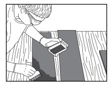
**7.** Apply a second coat of adhesive to two strips of lagging. Be sure to apply adhesive to the edges of the lagging as well.
