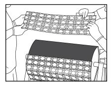
**9.** Place the second strip of lagging against the first, taking care to ensure there are no gaps between the lagging. This may require additional stitching between strips to remove any gaps. Repeat the tamping and stitching process in Step 8 to remove air gaps from the applied strip.
