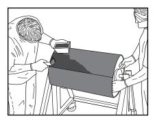
**6.** From the perpendicular line, apply a second coat of adhesive to an area slightly greater than two strips of lagging.
